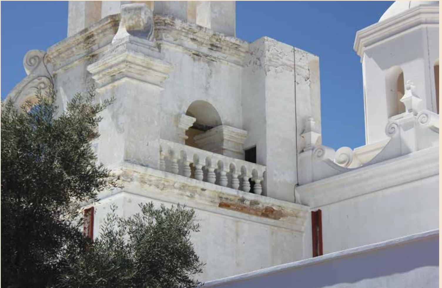
*The north side of the East Tower shows mold damage & broken cornice*
