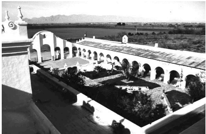
East Additions from Roof Top
