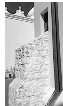
Rock Buttress West Wall
