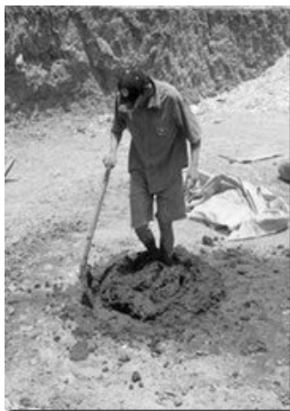
Mixing Adobe for bricks
