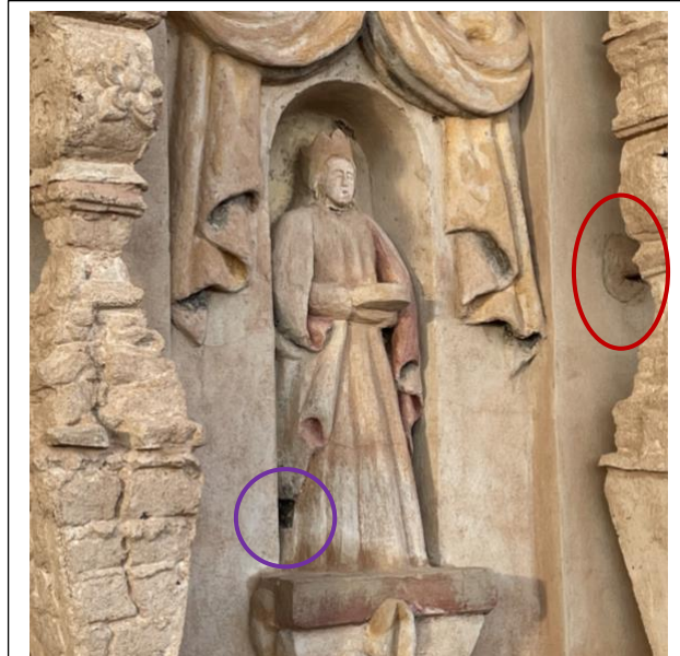
Saint Lucy on the right side of the retablo façade flanked by two replica estípites, which are held in place by metal reinforcements. The small black square on the lower right side of her dress is a test area where the plaster was removed to reveal the original coloring. Preservation work began on the façade in spring, 2024.
