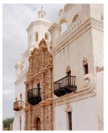
The three balconies on the front of the Mission are reproductions and date from different eras; two were built as replacements in the 1950s, one was built as part of the restoration of the West Tower in 2007. All are in very different states of repair.
