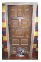
This door, located between the Nave and the ground floor room of the East Tower is likely the oldest of San Xavier's woodwork and possibly originating from Mexico. It is in use daily and has many condition issues, including some created by failure of the original hinge hardware.
