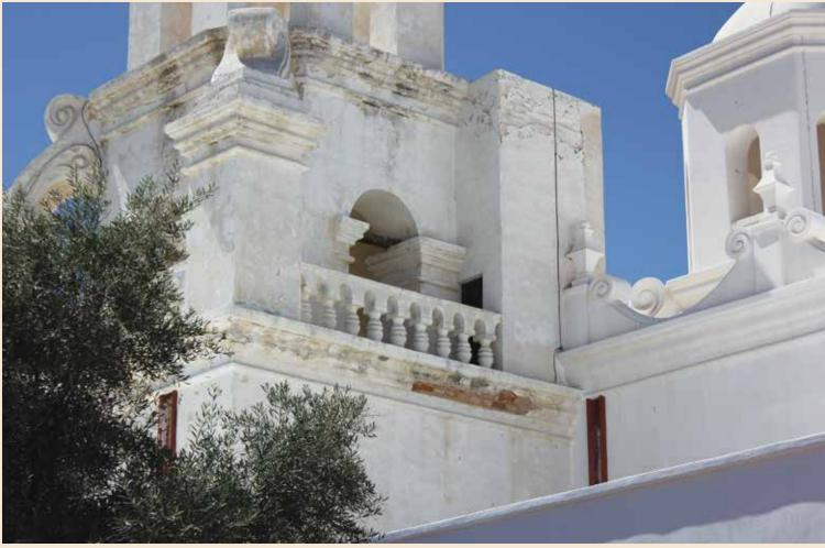
The north side of the East Tower shows mold damage & broken cornice
